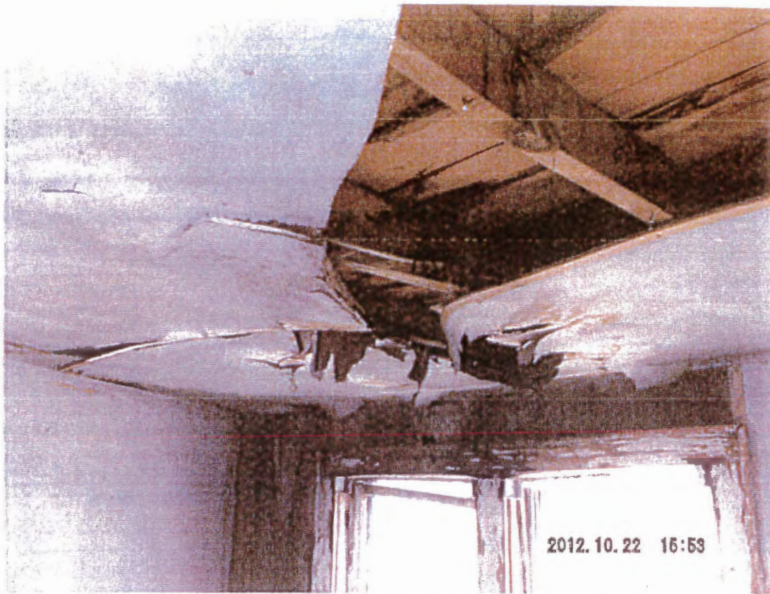
Picture showing water damage to sheet rock and roof members
