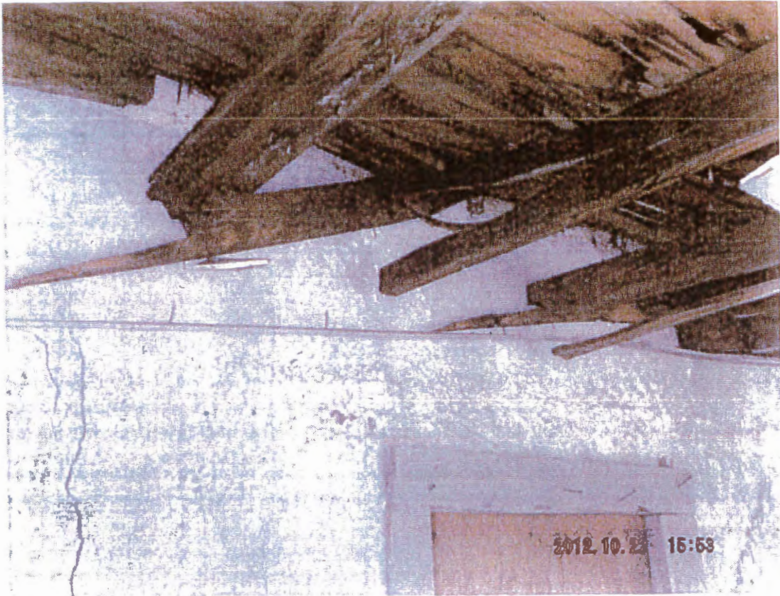
Picture showing failure of roof members
