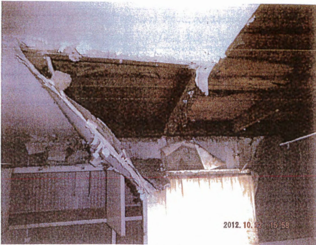
Picture showing water damaged sheet rock
